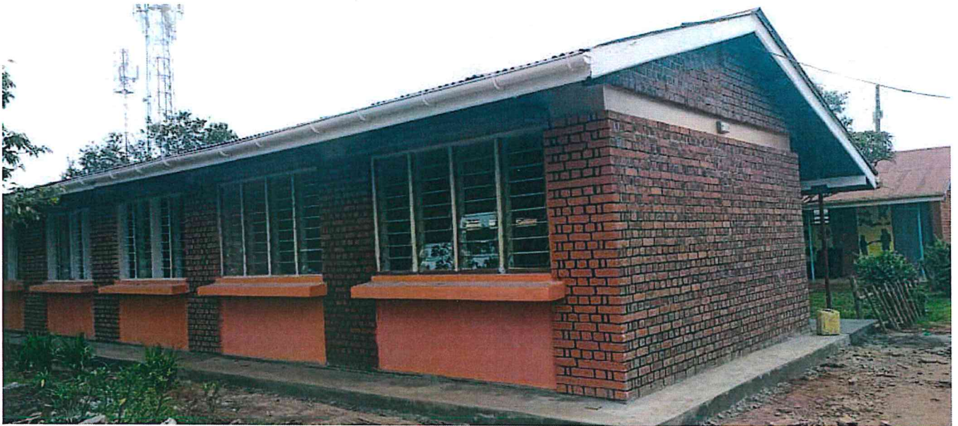
Figure 29: Showing Classroom block for Ntinda school for the deaf after renovation
