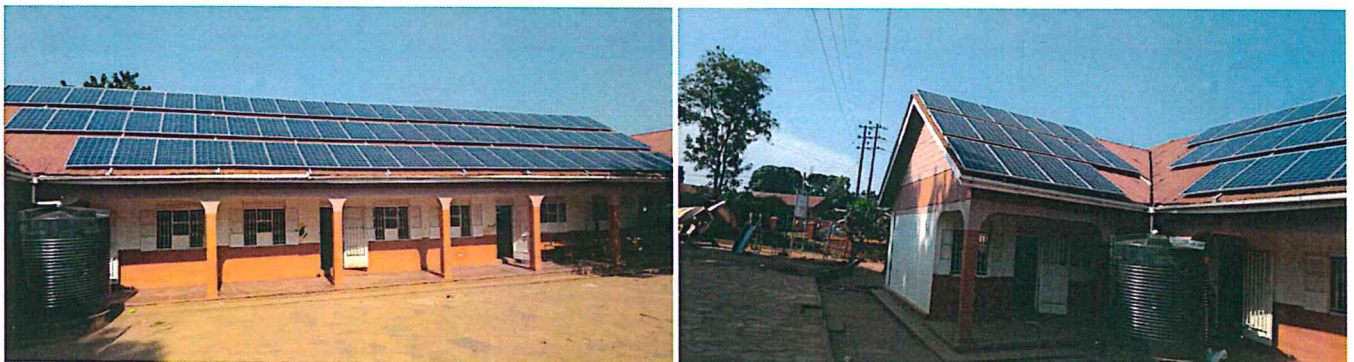
Figure 30 &31 showing Solar PV Installation works at Mulago school for the deaf
