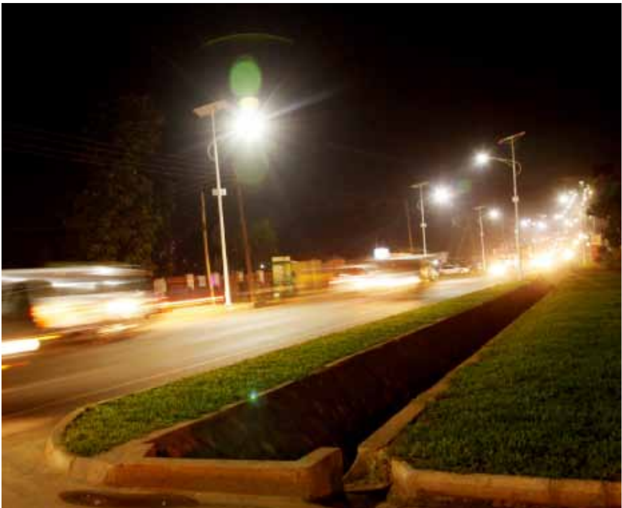
Kabakanjagala one the city roads constructed to enhance city mobility
