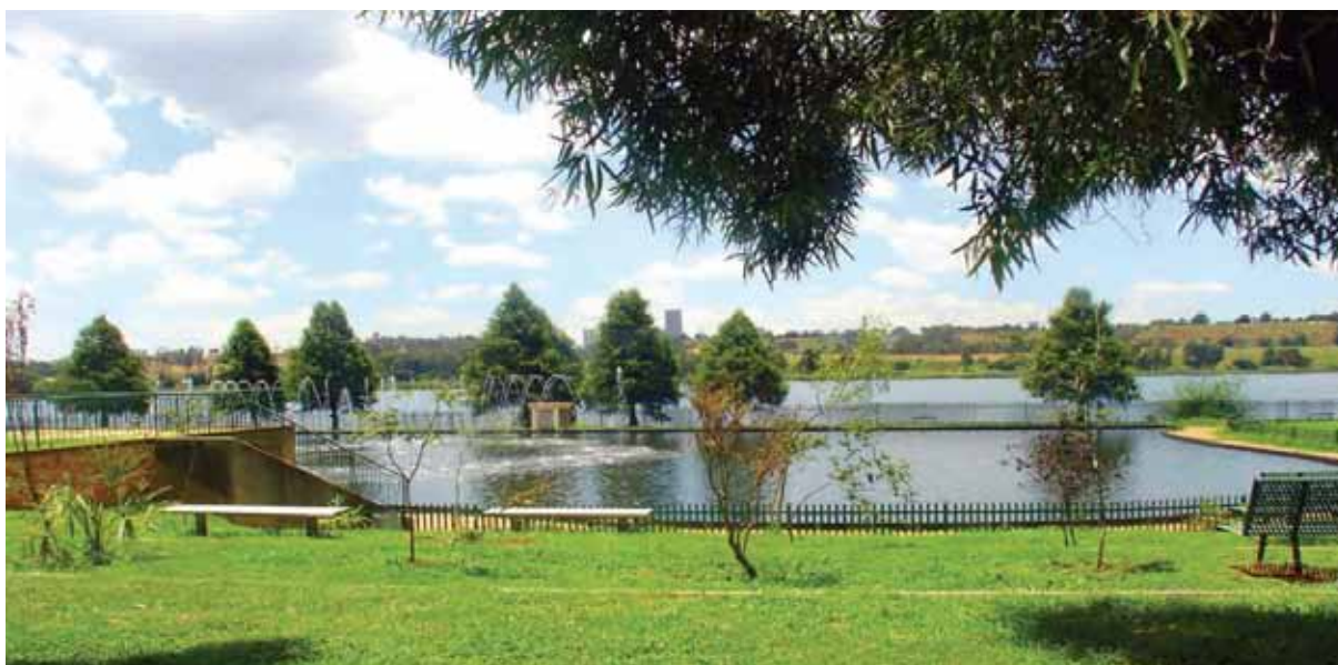
Watershed integrated with a community park to be promoted in many low lying areas that are vulnerable to flooding
