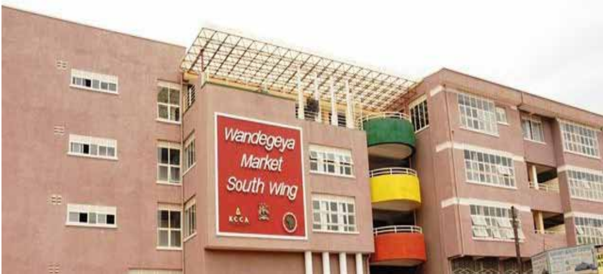
Wandegeya market constructed with financial assistance from ADB (2013)
