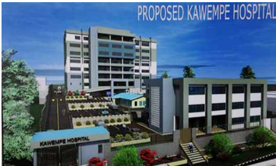
The Proposed Kawempe Hospital under construction with funding from ADB
