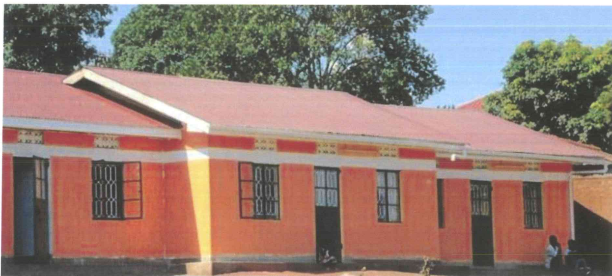
Renovation of staff quarters St. Mbaga Tuzinde Kiwatule
