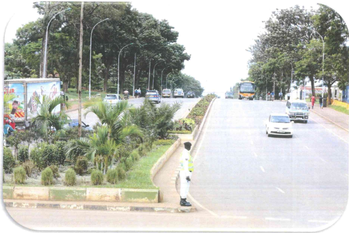
Section of Jinja Road Kampala (Central Division) reconstructed 2014/15
