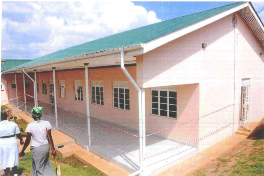
One of the recently refurbished blocks at Kitebi Health Centre Kampala
