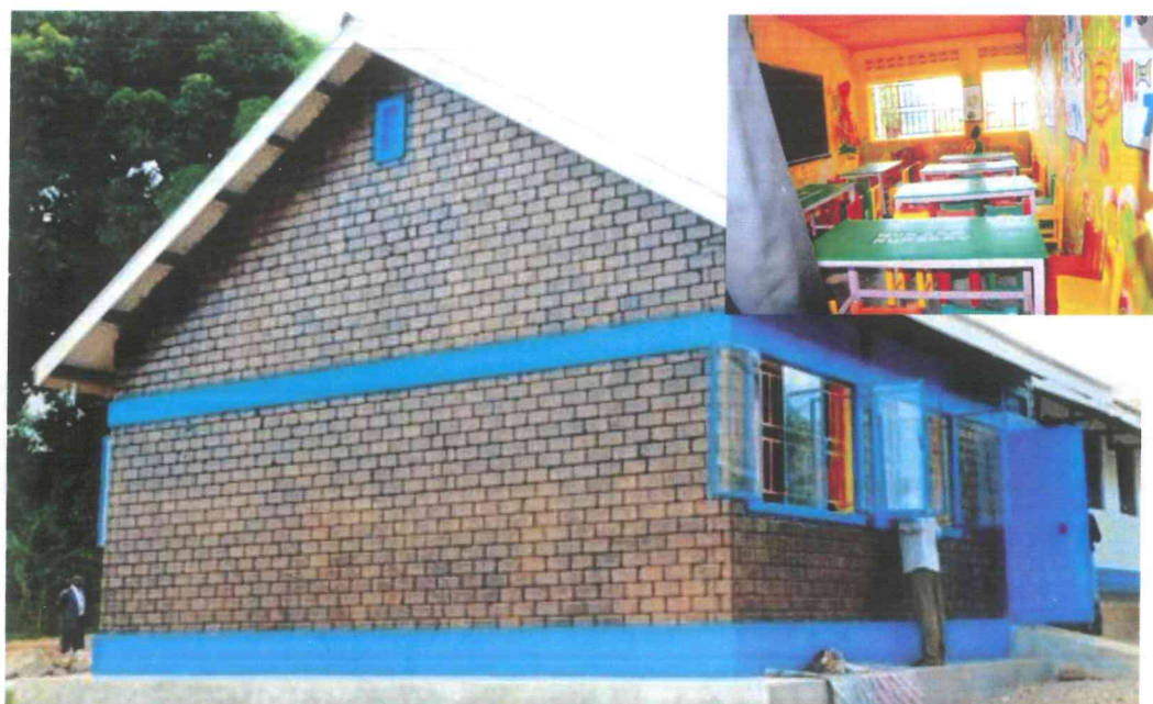
Nursery classroom block at Bukasa Primary School (Inset Inside the class)
