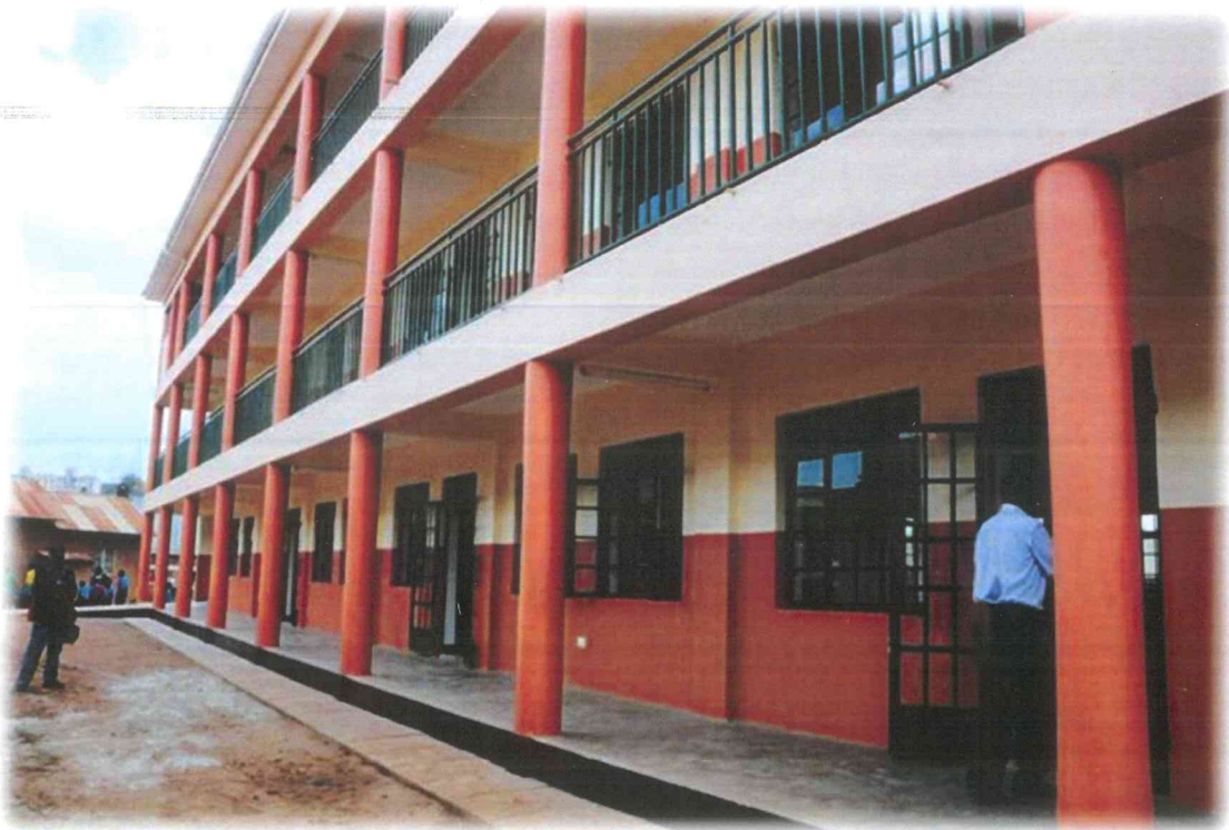
9 classrooms block constructed at KCCA Kamwokya Primary School
