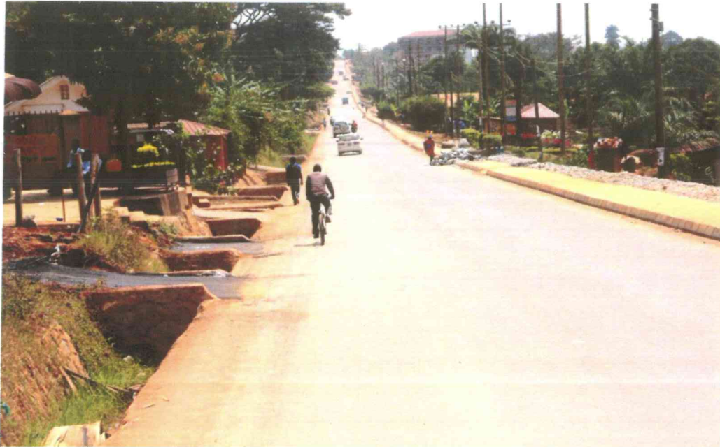
Construction works on Mutundwe road in Lubaga Division
