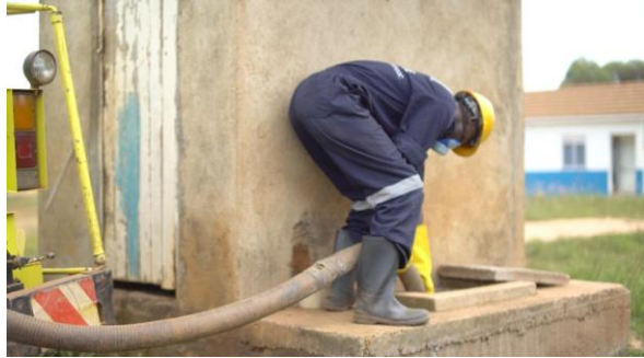
Figure 6: Safe Emptying of a lined toilet
