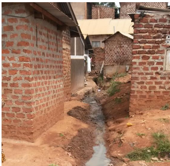
Figure 9: Toilet and Bathroom waste flowing into drains
