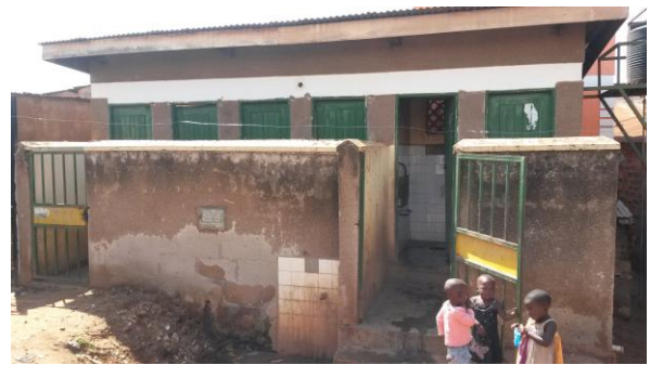
Figure 8: Community toilet in Kisenyi
