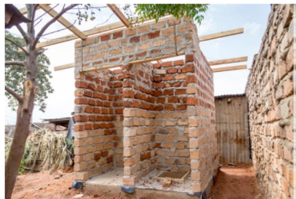
Figure 5: Lined facility under construction
