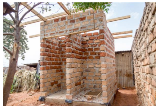
Figure 5: Lined facility under construction
