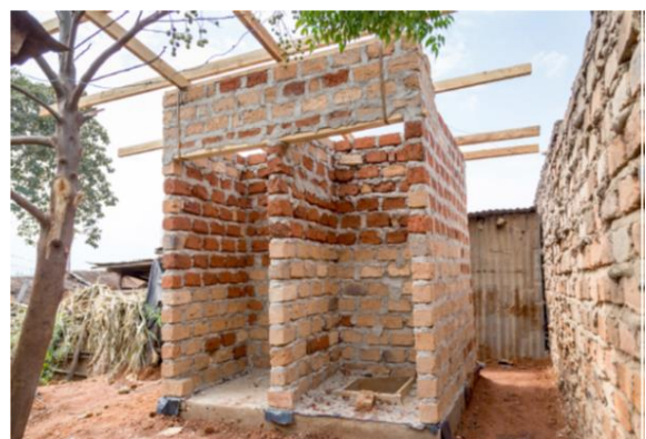
Figure 5: Lined facility under construction
