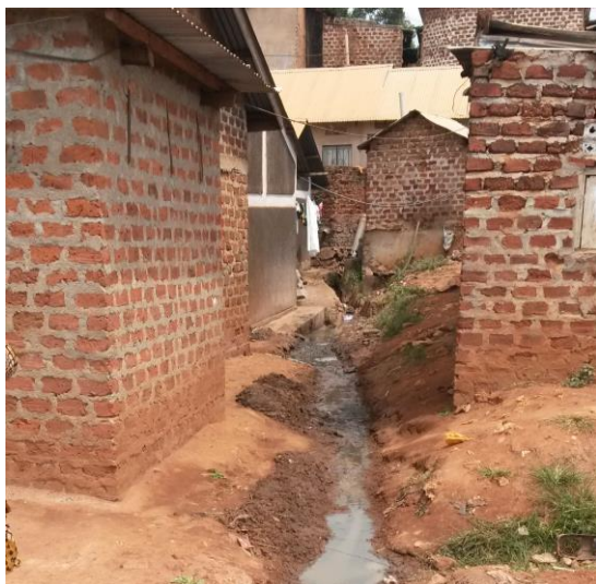
Figure 9: Toilet and Bathroom waste flowing into drains
