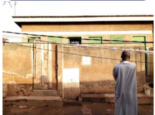
Figure 8: Community toilet in Makerere
