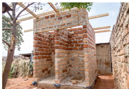
Figure 5: Lined facility under construction
