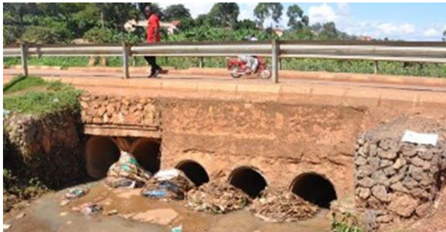
Figure 2-51: Kansanga Primary channel – Upstream culvert headwall Hanlon Road Crossing
