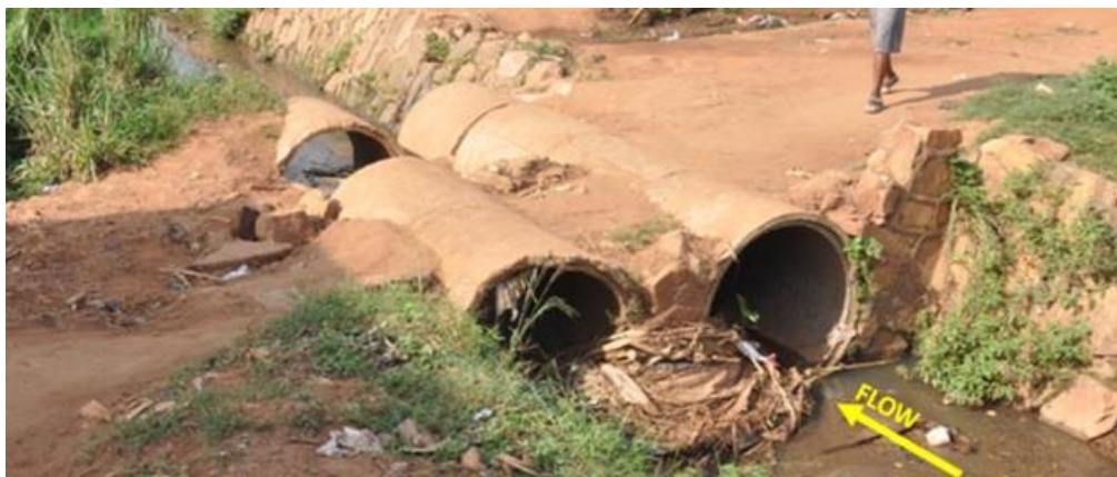
Figure 2-18: Type B Culvert – located at about Chainage 0+180m
