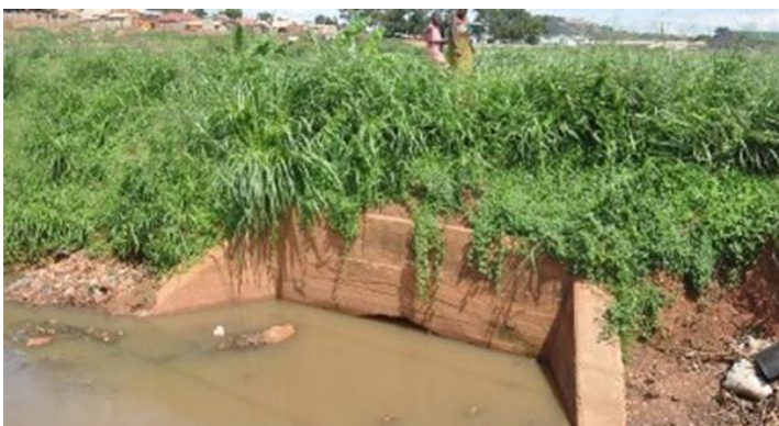
Figure 2-67: Kinawataka Primary channel - downstream headwall to rail line culvert
