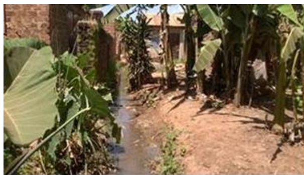
Figure 2-6: Typical unlined section along the channel
