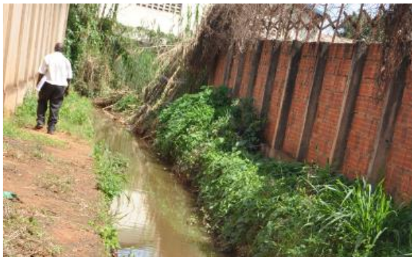
a) Boundary walls constructed with minimal land for drainage.
