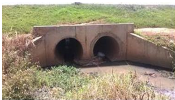
Figure 2-10: Channel draining through Northern bypass culvert with high invert level causing stagnation
