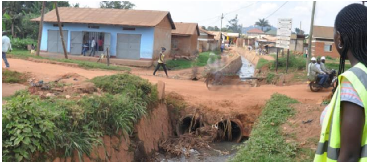
Figure 2-29: Upstream Headwall to Jakana Road Culvert
