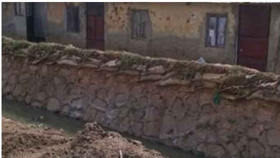
Figure 5-6: Sandbags used as flood barriers along a section on Secondary 8
