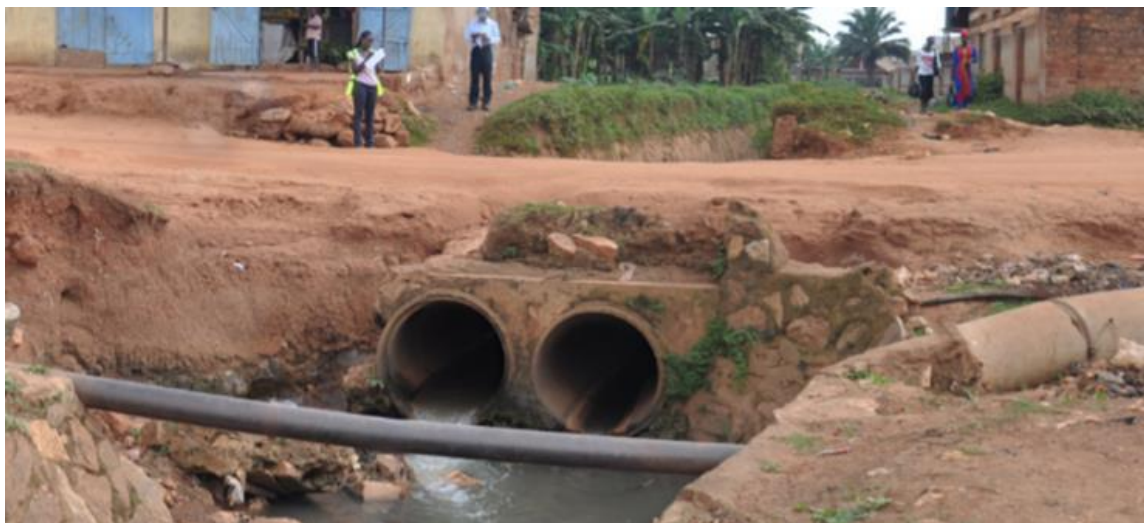
Figure 2-30: Downstream outfall from Jakana Road Culvert
