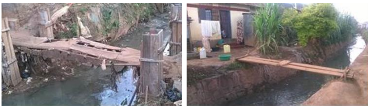
Figure 7-23: Unsafe drainage channel crossings typical in the dense residential areas
