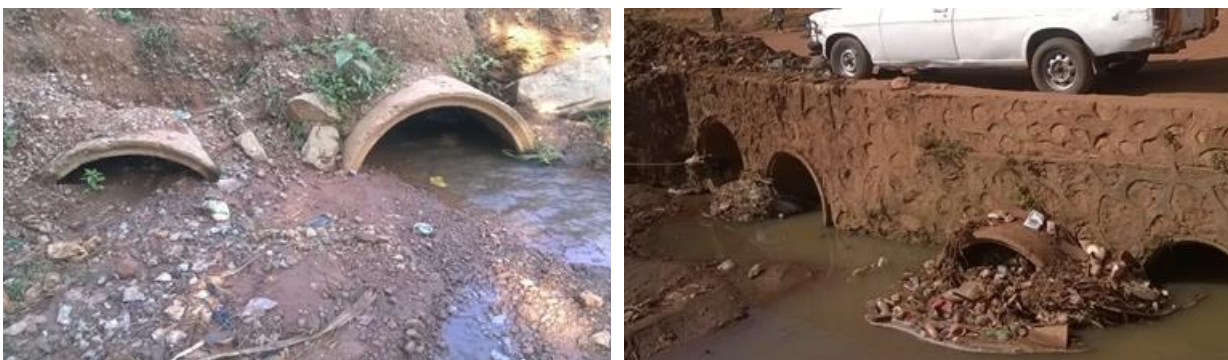
Figure 2-42: Blocked culverts by grit (left) and garbage (right) along the channel
