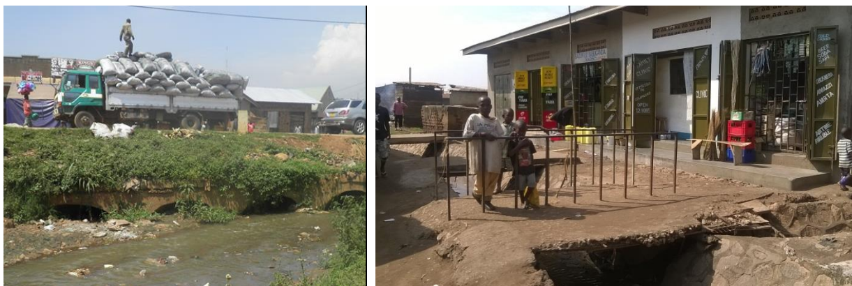
Figure 7-6: A failed culvert crossing to be improved along busy road - Secondary 10, Lubigi (L) and a channel crossing (R)
