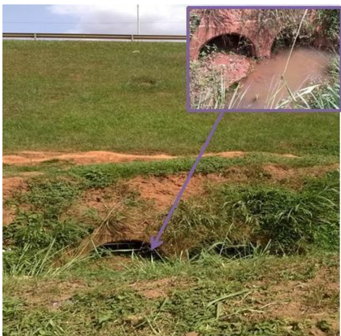
Figure 2-47: Blocked culvert below Northern bypass Bukoto-Kisaasi flyover
