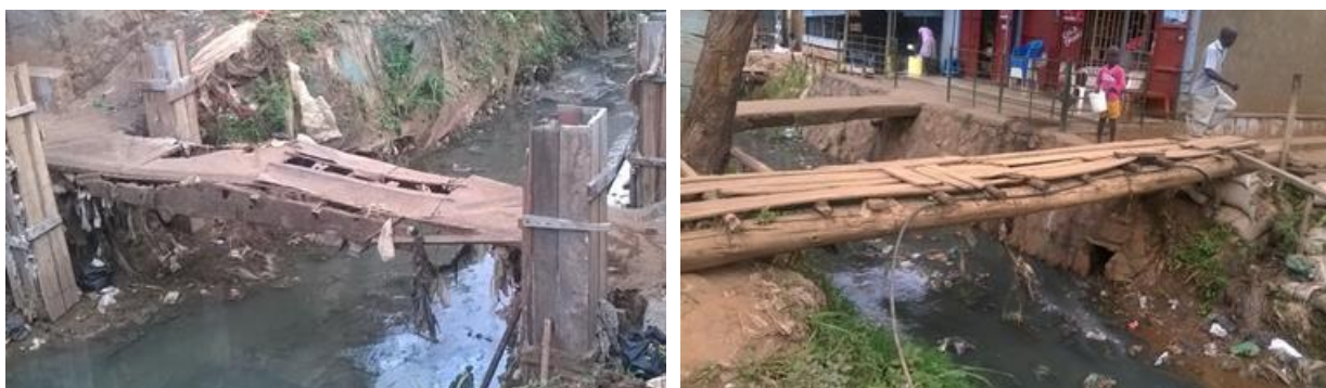
Figure 2-14: Improvised channel crossings made of scrap metal (left) and timber (right)
