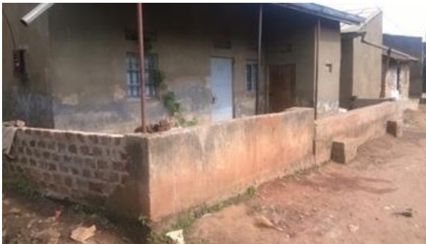
Figure 5-4: Typical example of flood barrier constructed around a house
