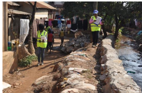
b) Typical example of channel bed higher than surrounding land
