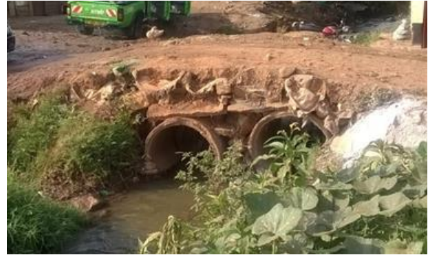
Figure 2-45: Improvised culvert at one section along the channel
