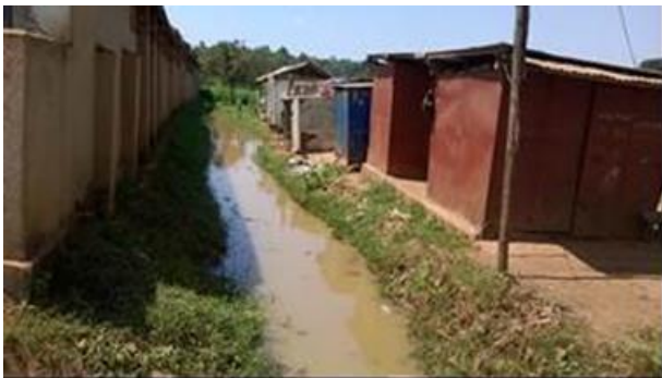
Figure 2-3: Natural lining typical of entire Channel length
