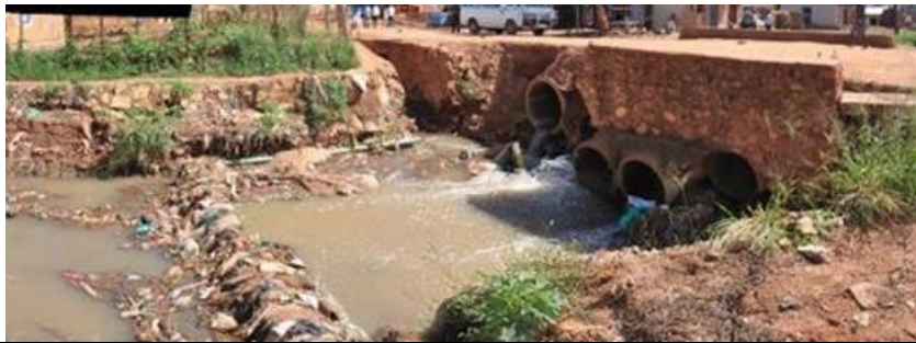
Figure 2-57: Kansanga Primary channel – Downstream culvert headwall Gogonya Road crossing
