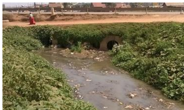
Figure 2-39: Clogged culverts at the Northern bypass before draining into Primary 2
