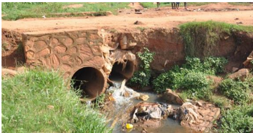
Figure 2-20: Downstream headwall for unnamed road culvert at about chainage 0+580m
