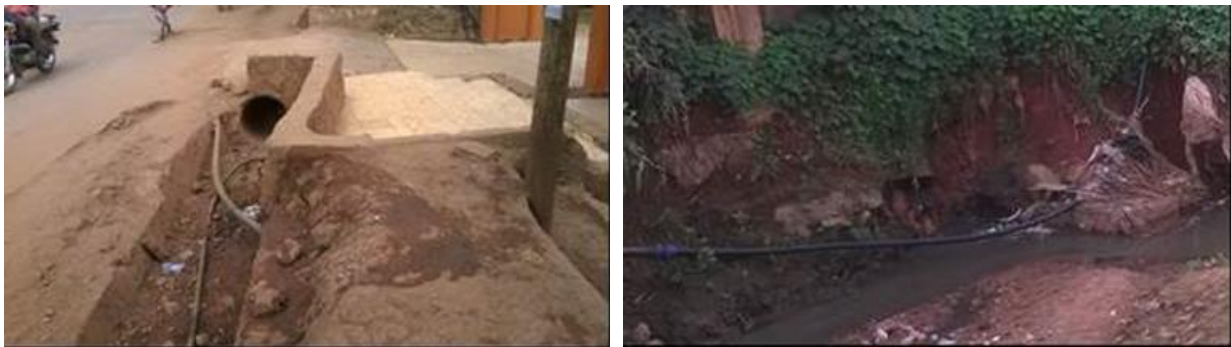
Figure 7-4: Water pipes running through sections of drainage channels
