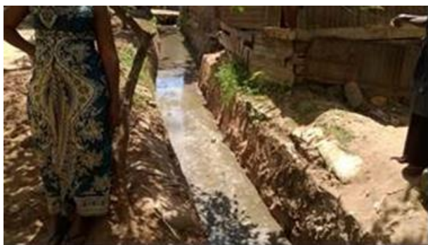
Figure 2-5: Typical masonry lined channel section between residential houses
