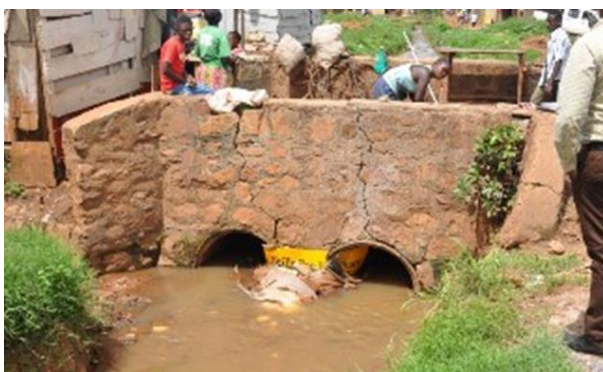
Figure 2-74: Kinawataka secondary channel 2 –upstream headwall for lane crossing
