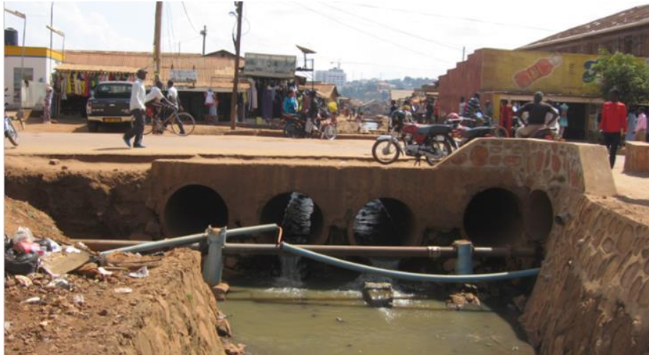
Figure 2-33: Downstream Headwall / Outfall to the Nabweru Road culvert
