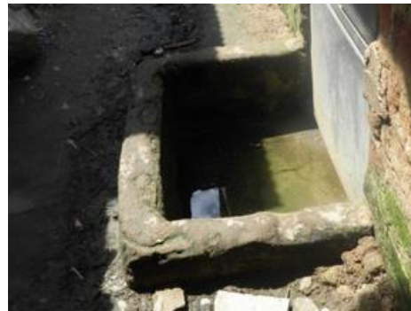
Figure 5-5: Typical example of flood barrier constructed outside a front door
