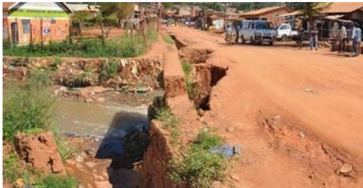
Figure 2-58: Kansanga Primary channel – Collapsed state of downstream culvert headwall
