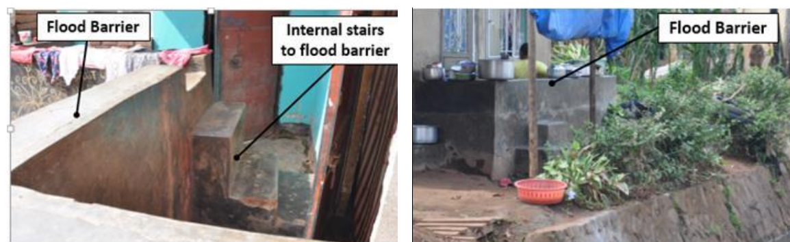
Figure 2-15: Flood indicators – barriers to homes and buildings to keep floodwater out.
