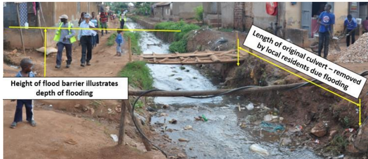
Figure 2-23: Chainage at about 0+970m - culvert causing flooding removed by local residents
