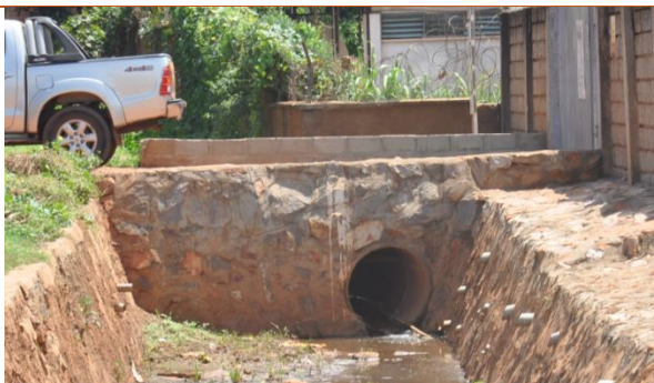
c) Small capacity culverts for access to industrial complexes
