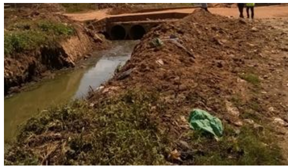
Figure 5-38: Silt dredged out of channel heaped along the edge
