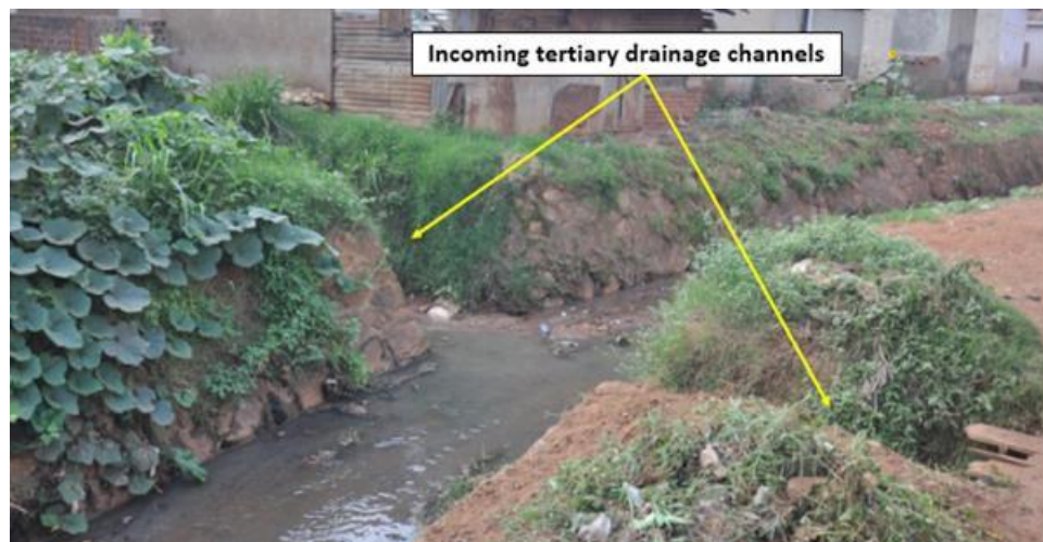
Figure 2-24: Typical of the many tertiary channels connecting to the secondary channels
