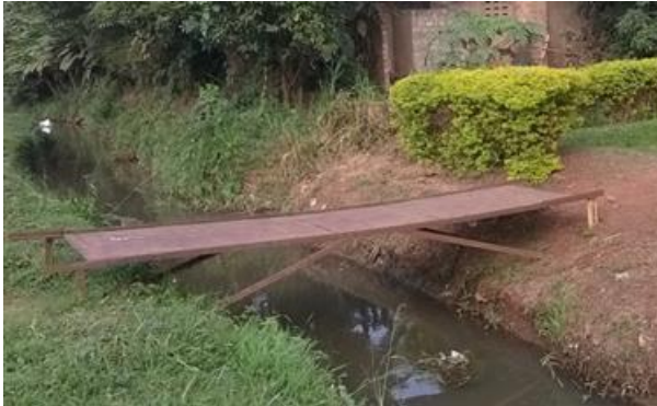
Figure 2-44: Earth lined section typical of the channel length
