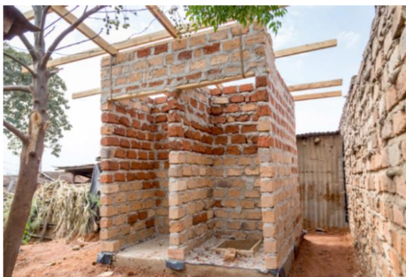
Figure 5: Lined facility under construction in Kamwokya
