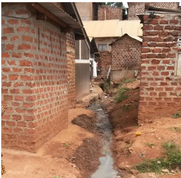
Figure 9: Toilet and Bathroom waste flowing into drains
