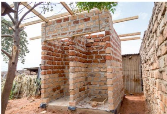
Figure 7: Lined facility under construction
